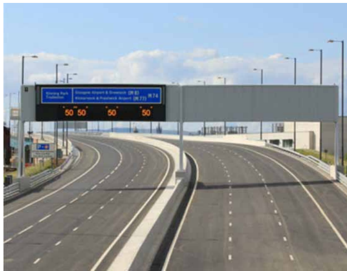
All-purpose gantry variable message signs on M74 extension.
